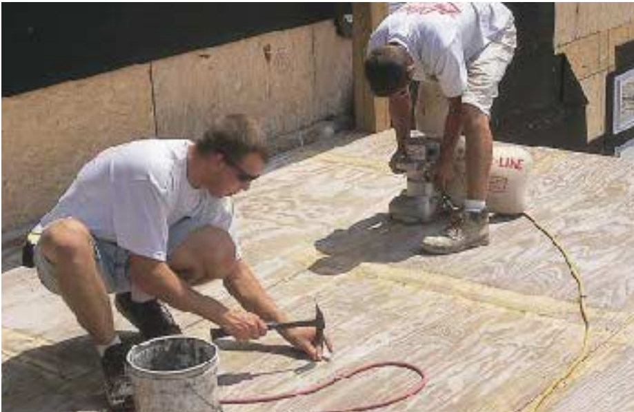
Figure 1. Prep work begins with setting nails and sanding all joints and edges in the tongue-and-groove plywood (above). Trowel-on floor filler is used to smooth any imperfections and to bridge any gaps in the seams and butt joints (right).
