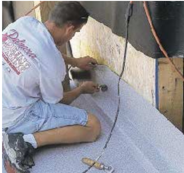
Figure 4. On the job shown here, Duradek was used as through-wall flashing for brick veneer cladding. The membrane covers the brick below and runs up the house wall and into the door opening. The remaining courses of brick were laid directly on the membrane, which directs any water trapped behind the brick onto the deck.
