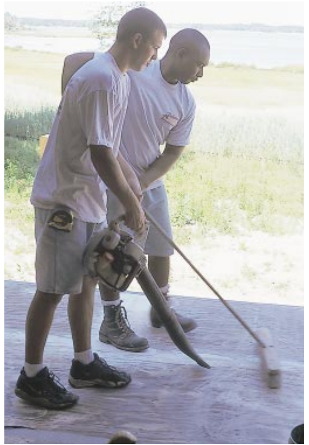
Figure 2. The crew smooths the dried patching compound using a light-grit paper in a palm sander (above). A once-over with a broom and a leaf blower clears the deck of any wood chips, roofing granules, and other debris that could get trapped under the membrane (right).
