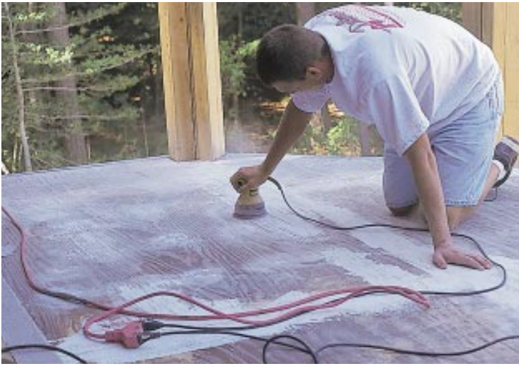
Figure 2. The crew smooths the dried patching compound using a light-grit paper in a palm sander (above). A once-over with a broom and a leaf blower clears the deck of any wood chips, roofing granules, and other debris that could get trapped under the membrane (right).
