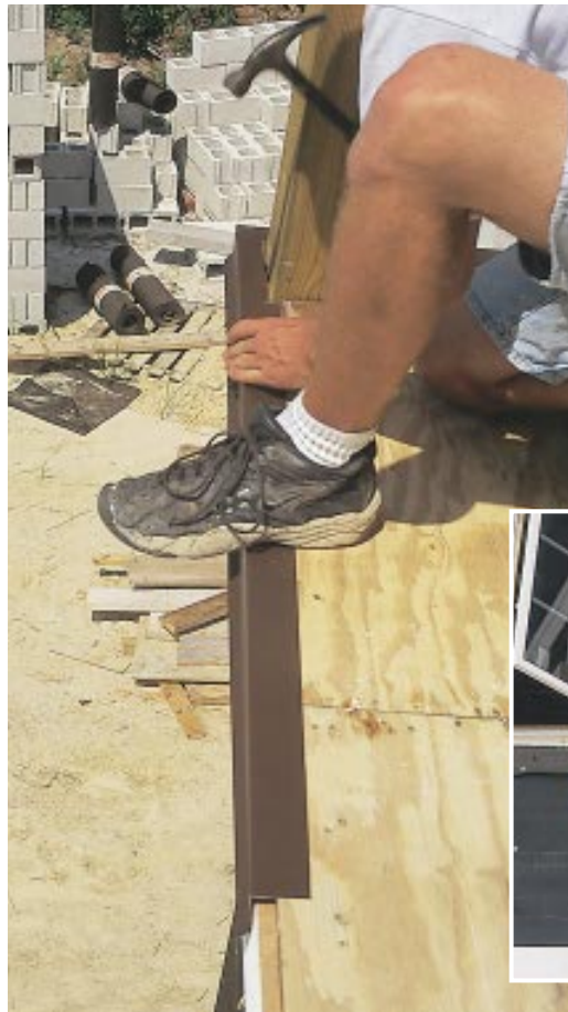
Figure 3. At the perimeter, the membrane is glued over a custom-bent metal drip-edge (left). To create a finished edge, the membrane is tucked under the kickout and capped with a vinyl trim strip (below).
