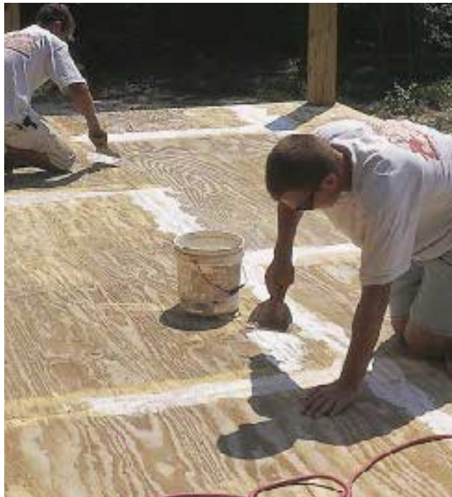
Figure 1. Prep work begins with setting nails and sanding all joints and edges in the tongue-and-groove plywood (above). Trowel-on floor filler is used to smooth any imperfections and to bridge any gaps in the seams and butt joints (right).
