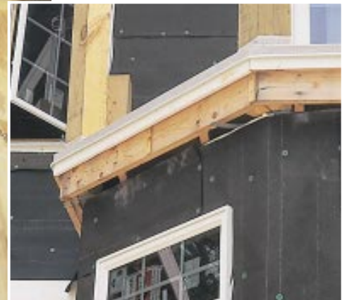
Figure 3. At the perimeter, the membrane is glued over a custom-bent metal drip-edge (left). To create a finished edge, the membrane is tucked under the kickout and capped with a vinyl trim strip (below).
